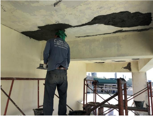
Staircase: Ceiling repair
