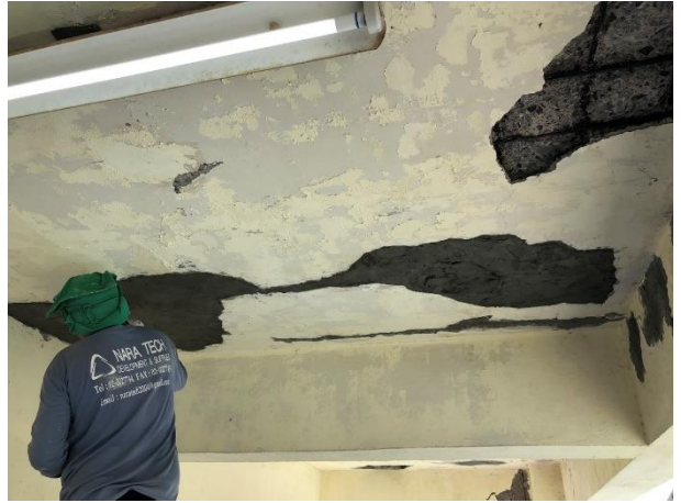
Staircase: Ceiling repair
