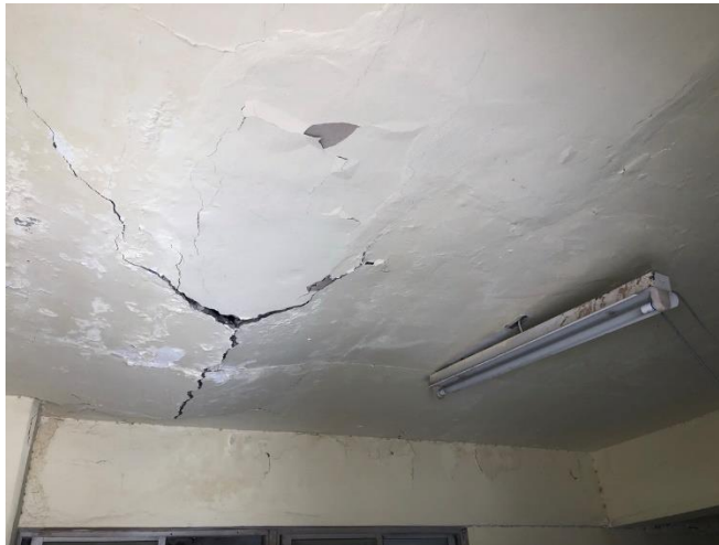
Staircase: Condition before repair
